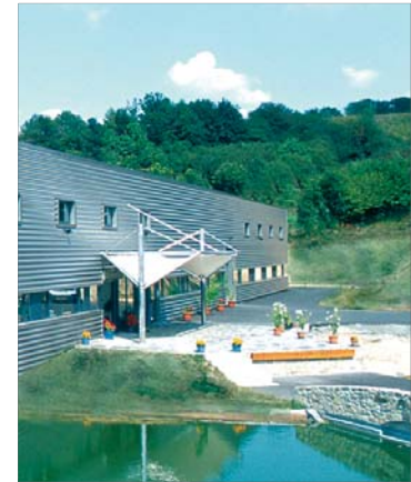
interscience R&D center and manufacturing plant
